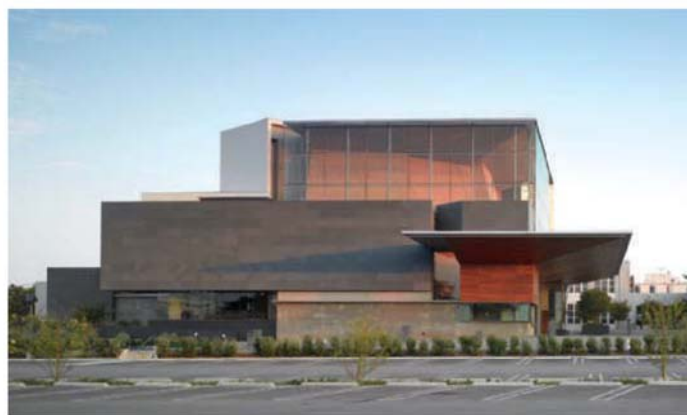
The theater's south elevation faces busy Santa Monica Boulevard.
